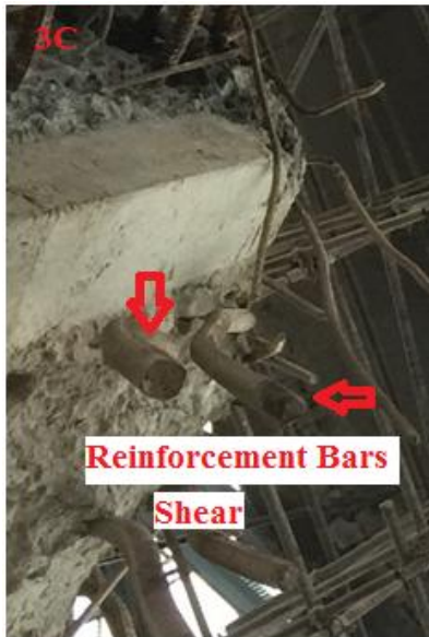
Figure 3a B C: Junction Of The Hopper And The Ring Beam
